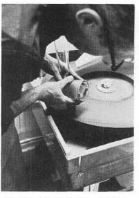
GLASS GRINDING OPERA-TION, using a flat cast iron grinding wheel with carborundum grit and water as the grinding medium, is performed in this photo by Bert DuMars.
